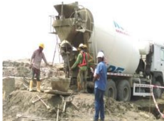
NDE Workers with PPE
