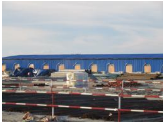
Beracades for keeping hazardous Materials
